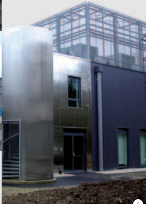
1. 2. 3. Power Station Pont-sur-Sambre - France
